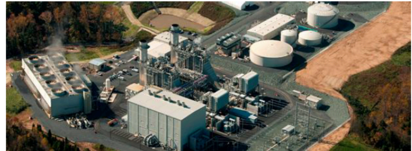
2. Dominion Virginia Power Bear Garden Power generating station, New Canton, Virginia, USA, 590 megawatt capacity
