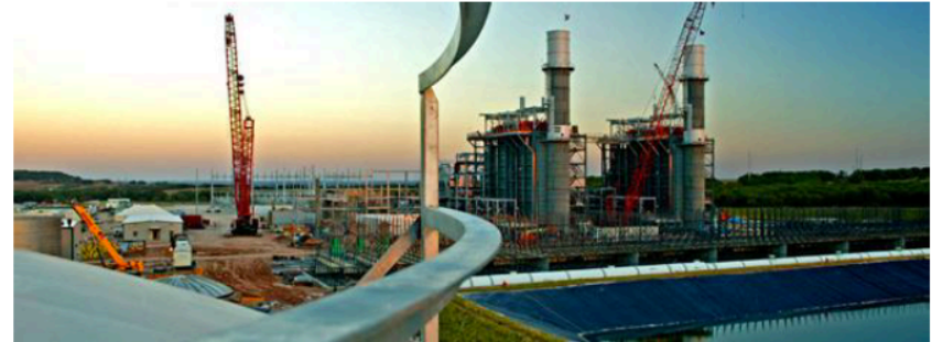
1. Brazos Electric Cooperative Jack County Gas-fueled power plant, Jacksboro, Texas, USA, 620 Megawatt capacity
