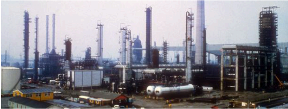
8. Antwerp, Belgium Refinery for Esso, 250,000 barrels per day
